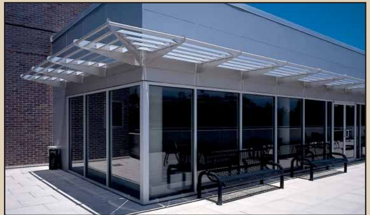
Architect: Rafael Architects | KSHB-TV
