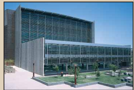
Architect: Bruder DWL
