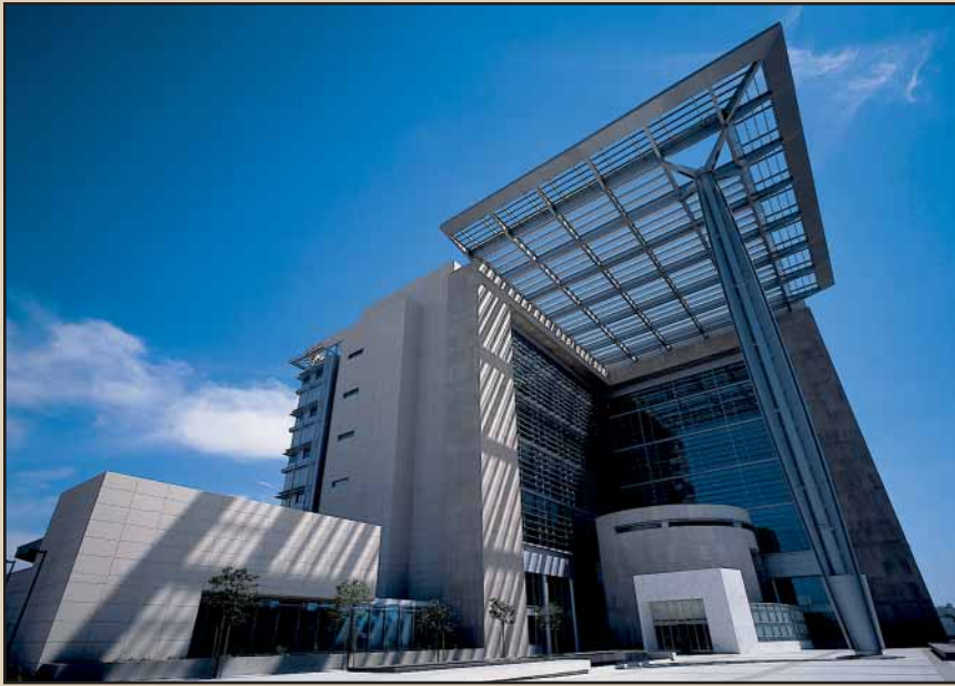
Architect: Cannon Dworsky/HCA and Langdon Wilson Las Vegas Courthouse
